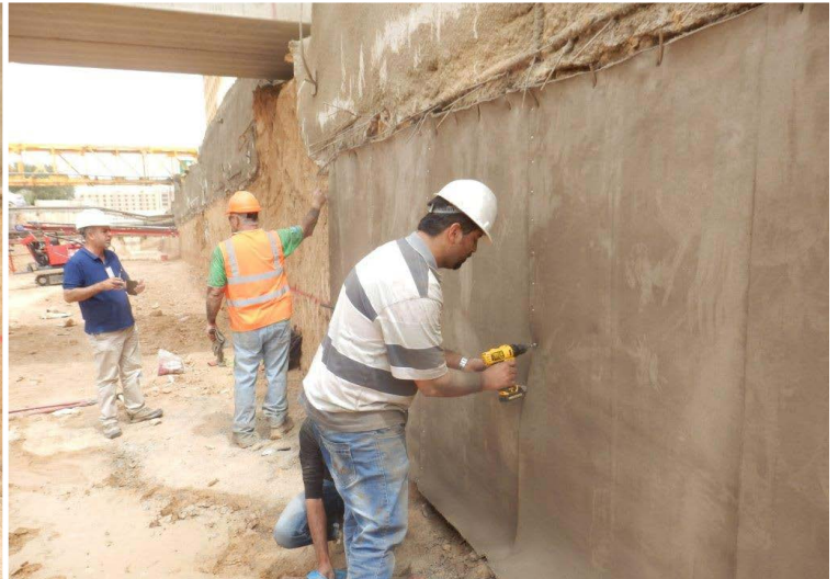
The joints being screwed
