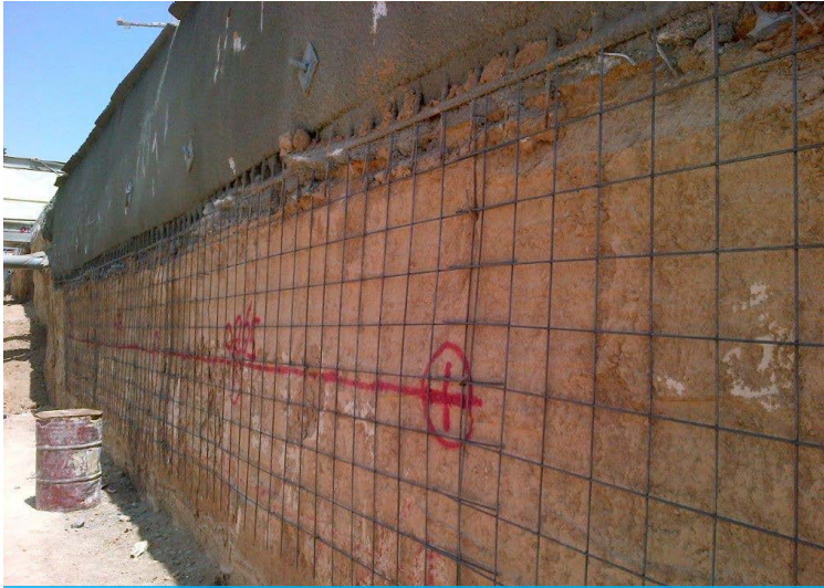
Mesh being sized up pre-installation
