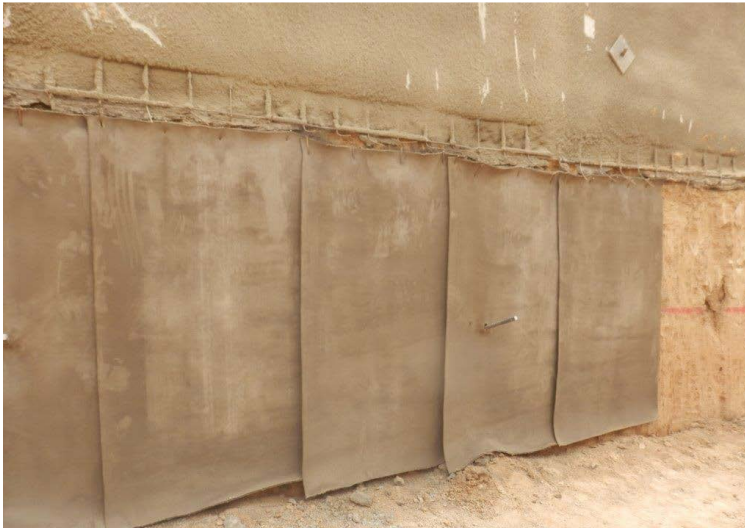
Fixed with soil nails
