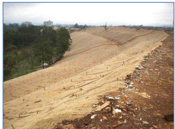
Slope with SoilSaver® jute pegged to surface
