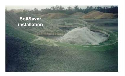
As with most outdoor sporting facilities there was a need for all-weather playing conditions or quick recovery after rain. To this end subsoil drains were installed in the bunkers, under greens and fairways of the golf course. **Kaymat U12** was used in all the bunkers to separate the subsoil from the bunker sand. It was also used in an unusual application, as temporary protection to the bunker sand stockpile.
