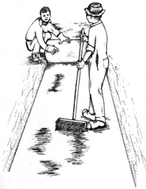
4. Place or roll out a suitable width of **Sealmac**, by hand, which will cover the affected area or crack. This is carried out immediately after the emulsion has been applied. The tack coat should reflect through the **Sealmac** upon pressure applied by fingertips. The **Sealmac** patch should not slide freely under pressure exerted by hand. Ensure that all creases and fishmouths are ironed out by using either a squeegee or the reverse section of a hard broom.
