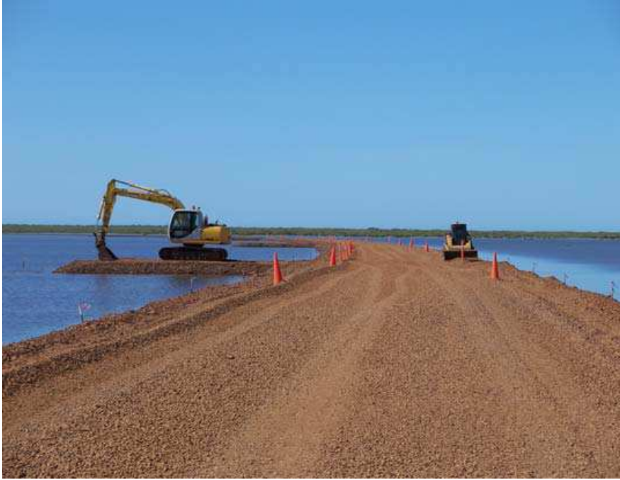
Construction of the temporary causeway
