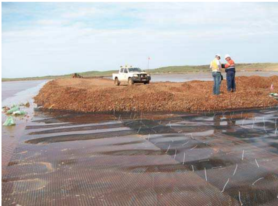
Tensor biaxial geogrid installation
