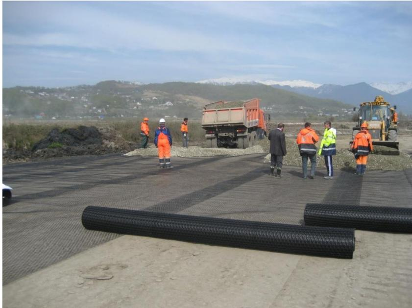
*Tensar TriAx® geogrid being installed at the coastal cluster sites
