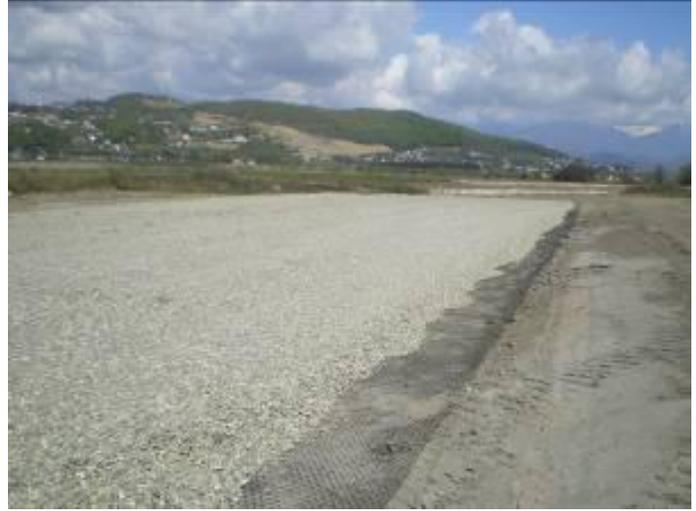
*Installation of the mechanically stabilised layer*
