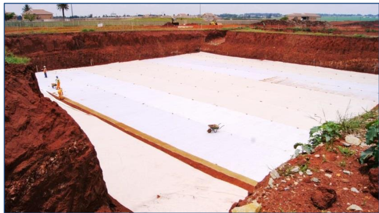
Rockgrid® PC laid at excavation depth
