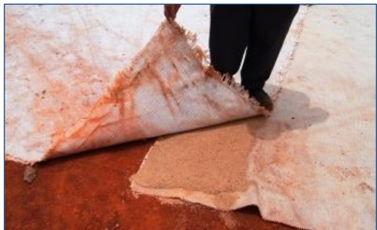
Rockgrid® PC 500mm overlap with riversand between the overlays to increase the friction angle between the layers
