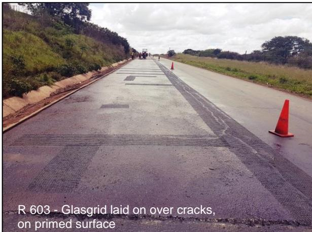
Typically, some causes of pavement cracking are loading, age hardening and temperature cycling. GlasGrid® paving reinforcement combines strength and elasticity for long-lasting performance and helps arrest this cycle of deterioration. It's the hidden strength in the road, reducing reflective cracking for years to come. The combination of high tensile strength and high modulus of elasticity at low elongation makes GlasGrid® stronger than steel in asphalt reinforcement applications.
