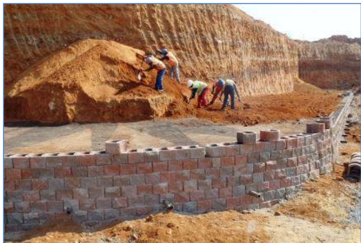
Miragrid GX 80/30 placed for reinforcement of the block wall
