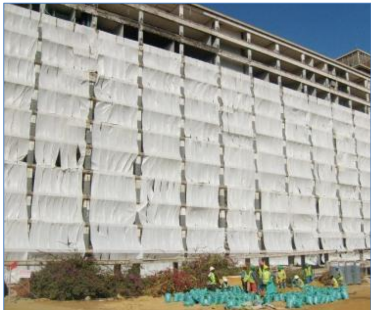
The 11-storey building ready for demolishing
