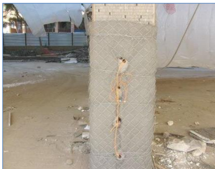
Each column was wrapped in bidim ® A10 to contain blast fragments
