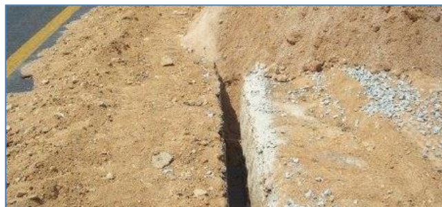
The drain is then backfilled with in suit soil
