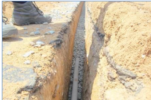
Aggregate is filled in around the Megaflo™ panel drain
