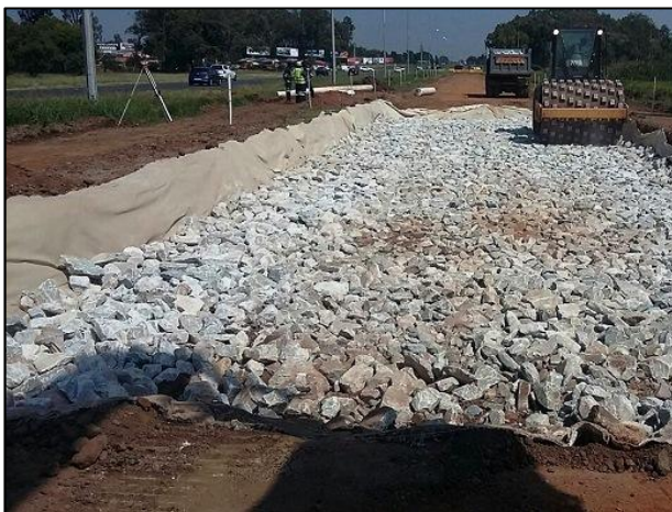
The Alternative: Crushed Rock and Geotextile (Expensive!)
