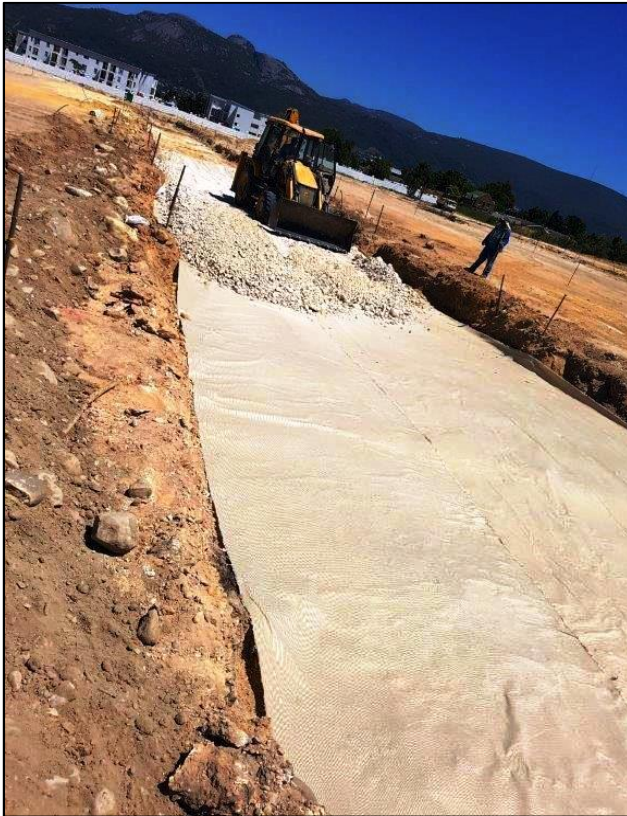
Installation of Sand Over Rockgrid® PC Geogrid
