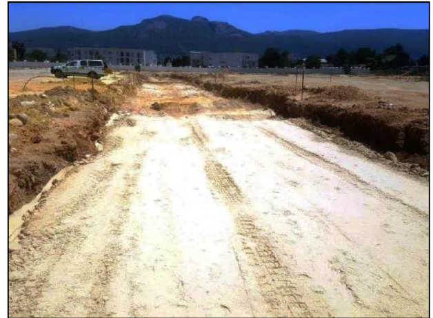
Sand Placed over Rockgrid® PC Geogrid
