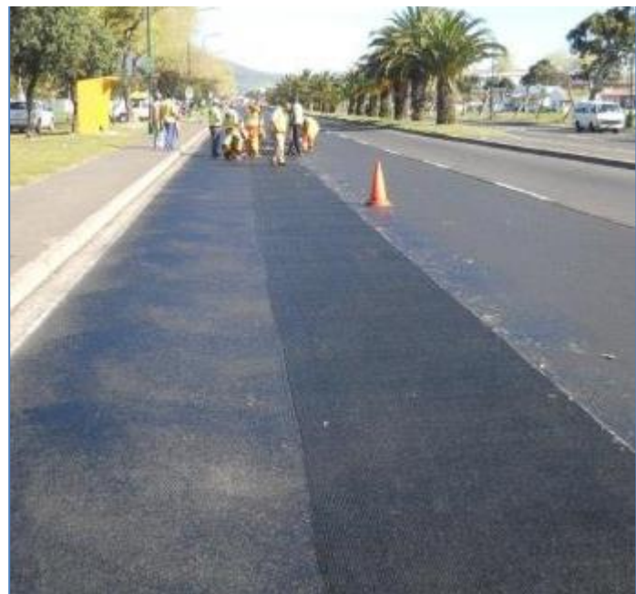
2 grades of GlasGrid were laid for the bus and outer lanes.
