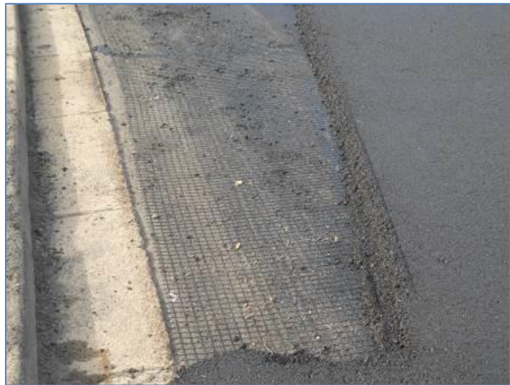
GlasGrid was laid between the levelling and surface layers of asphalt.
