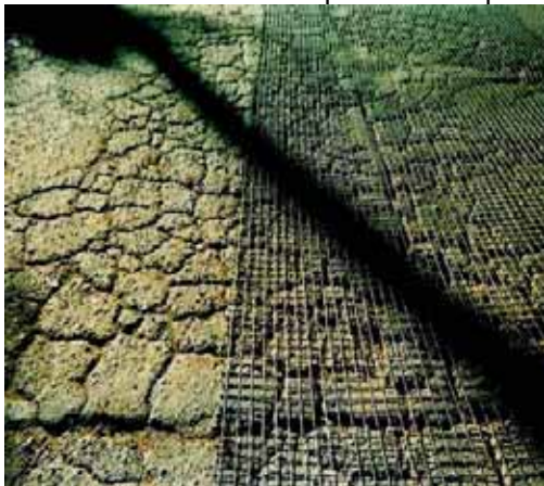
This photo shows the severely cracked road before rehabilitation.
