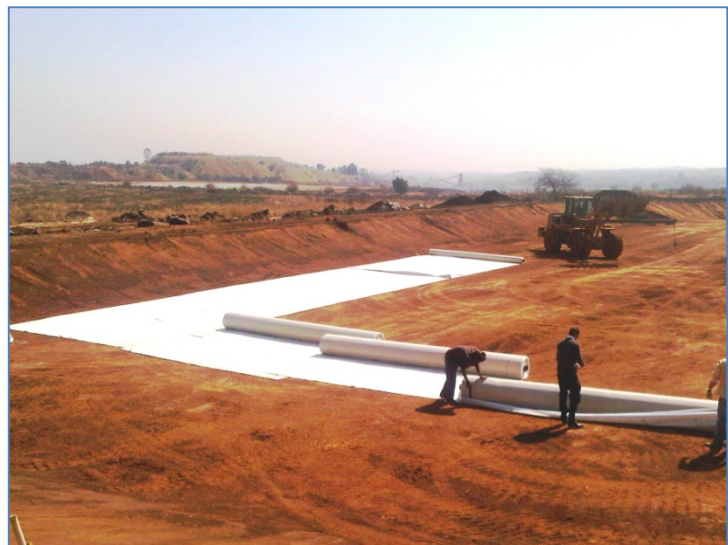
Laying EnviroFix® X800 on the base of the dam
