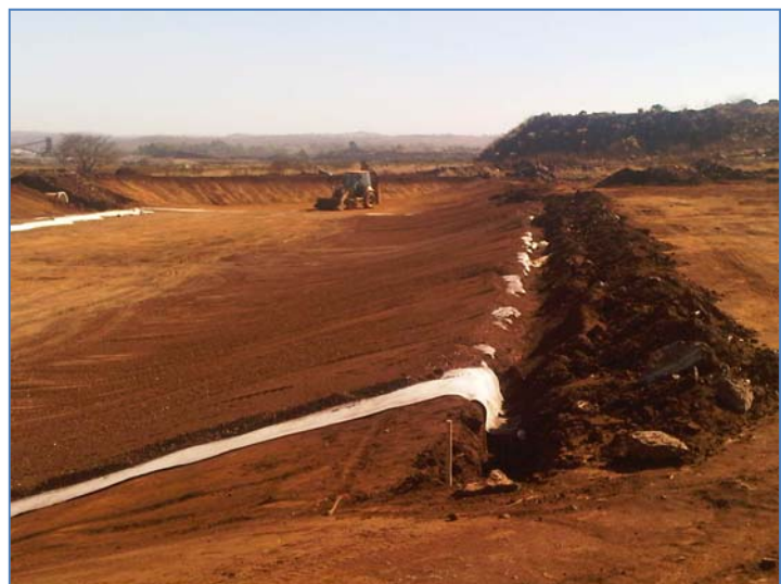
EnviroFix® X800 is secured in place in an anchor trench
