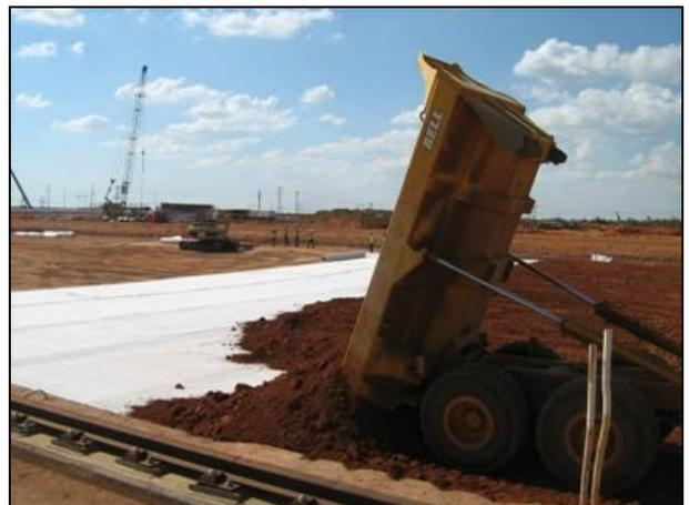
The GCL was placed by use of a spreader bar and a layer of 300 mm-compacted soil was placed over it.
