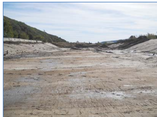
The re-shaped dam
