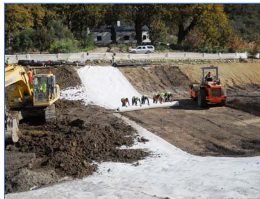
Laying Envirofix GCL over the prepared surface
