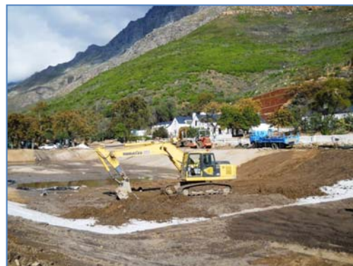
The layers - prepared surface, Envirofix , cover soil
