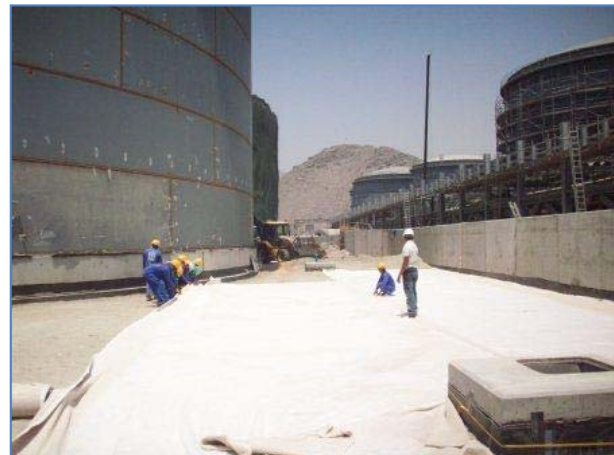
EnviroFix ® was manually laid due to the pedestals.
