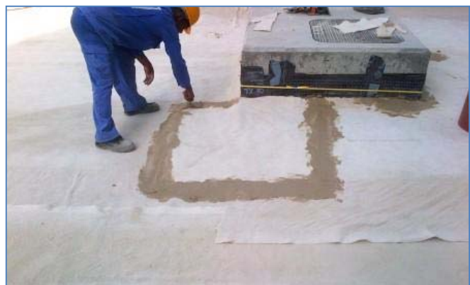
The many edges were sealed with Bentonite paste.
