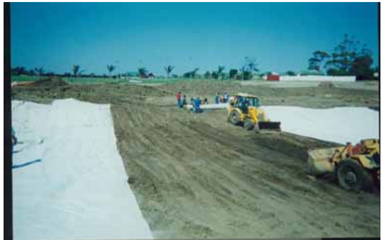
Laying of Enviromat™ X800 GCL
