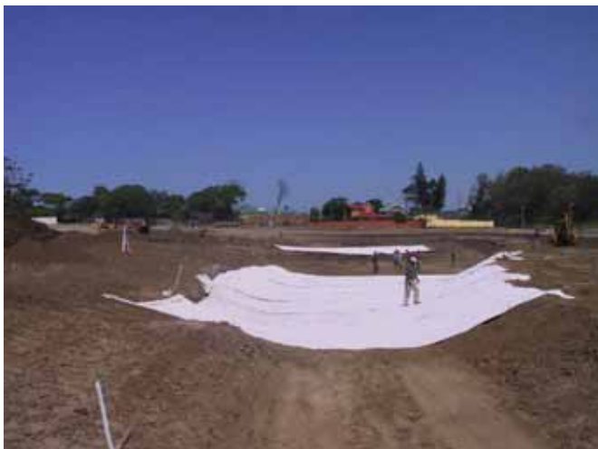
Laying of Enviromat™ X800 GCL
