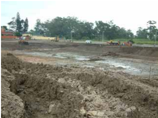
Excavation of water feature dam
