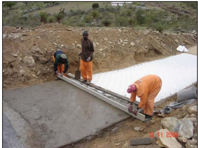
Base preparation, Multi-Cell panels tensioned to side forms, concrete placement and screeding
