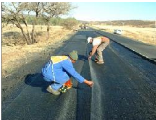
Km 42 946 – GlasGrid® 8501 installation, 2003
