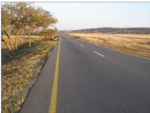
Km 42 946 – GlasGrid® 8501 performance, July 2008
