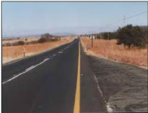
Km 16.28 – GlasGrid®/Sealmac® installation, 2003
