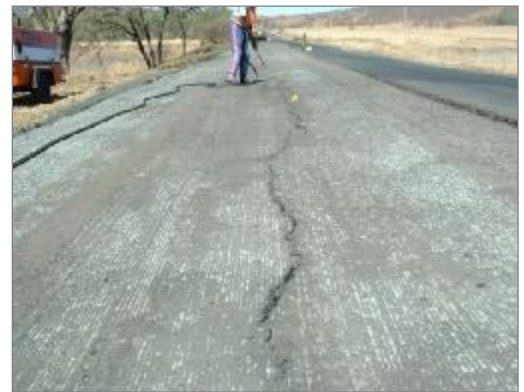
Km 42,946 – Crack under milled surface, 2003
