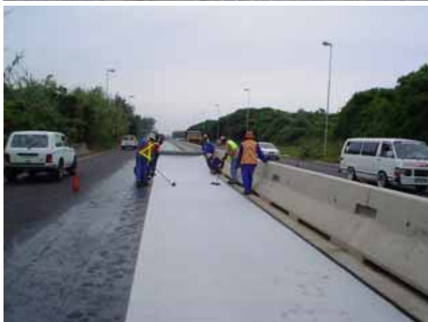
1. Condition of existing surface – 27 February 2004 2. Roll out Sealgrid into broken Colpave™ tack coat. 3. Broom out bubbles, folds and creases. 4. Roll with PTR.
