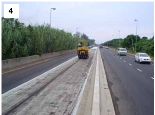
1. Condition of existing surface – 27 February 2004 2. Roll out Sealgrid into broken Colpave™ tack coat. 3. Broom out bubbles, folds and creases. 4. Roll with PTR.
