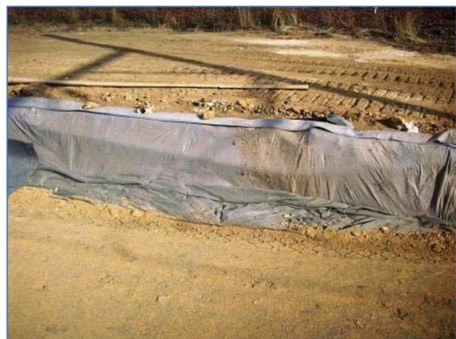
***Flo-Drain™** for subsoil drainage*
