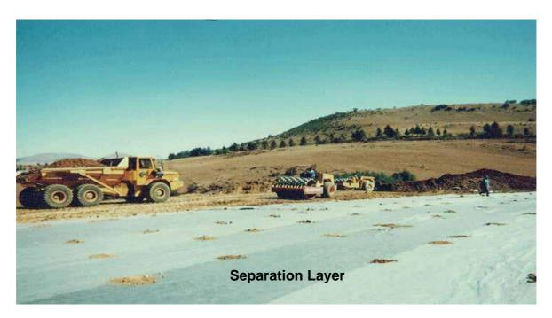
**Kaymat** is the ideal product for separation applications as it combines high strength and conformability with excellent transverse throughflow characteristics
