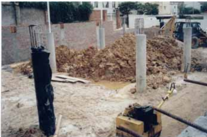
Above: Installation & compaction of sand layer Below: Isolated areas needed releveling
