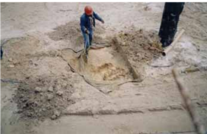
Above: Installation & compaction of sand layer Below: Isolated areas needed releveling
