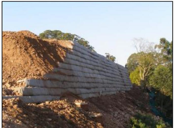
The design standards used were SANS 207 for the wrap-around wall and SABS 1200D for the earthworks. A simple base was constructed by benching 1200mm into the existing material, compacting and then levelling the surface. The wall reinforcement comprised tiebacks at 600mm lift intervals, ranging from 1500mm to 6000mm in length.
