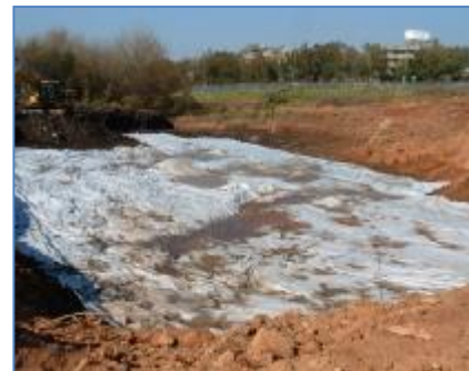
Installation of Rockgrid® PC geogrid
