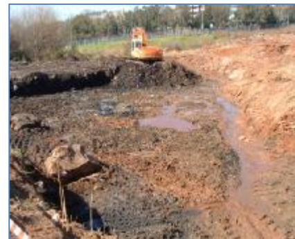
Removal of waste material
