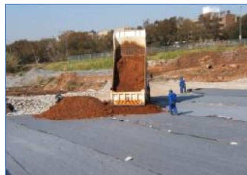
Applying backfill over the drainage/separation nonwoven
