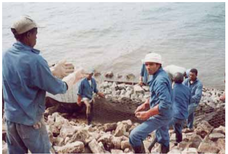
This type of construction is ideal for labour-based contracts.
