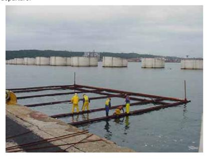
A Bidim A6 sock barrier was used between the caissons to prevent leakage of the sand fill behind the caissons from leaching out of the reclaimed area and into the harbour. Bidim A6 was also used as an inner lining on the fill side of the caissons as a further measure to prevent the sand fill from filtering out from behind the quay wall.
