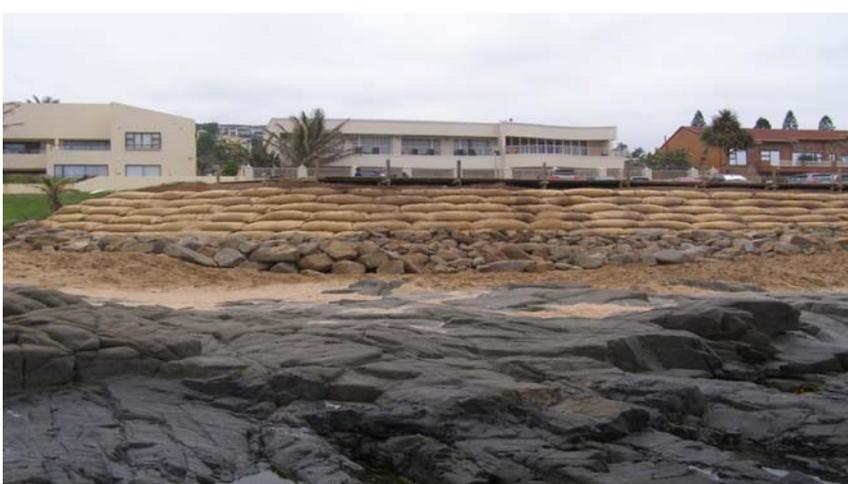
The design accepted for this project was a wrap around wall designed with Kaytech RockGrid® PC 100/100 geogrid and the Kaytech EnviroRock® Geocontainer® bags. Designed to protect the integrity of the base layers of the car park, the wrap around wall was installed from the face of the car park progressing under the car park. The EnviroRock® geocontainers were then designed in a stepped formation in front of the RockGrid® PC 100/100 wrap around wall to
