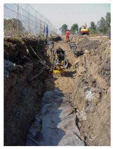
intersected at depths as shallow as 0.5m in places. created some difficult installation conditions as a stable dry foundation and excellent pipe bedding compaction is imperative. The this solution to problem involved the excavation of a further 300mm depth accommodate two additional. engineered layers.
