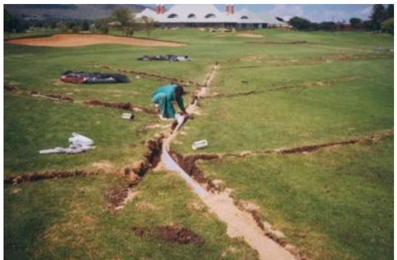
Placing of river sand backfill around MEGAFLO
