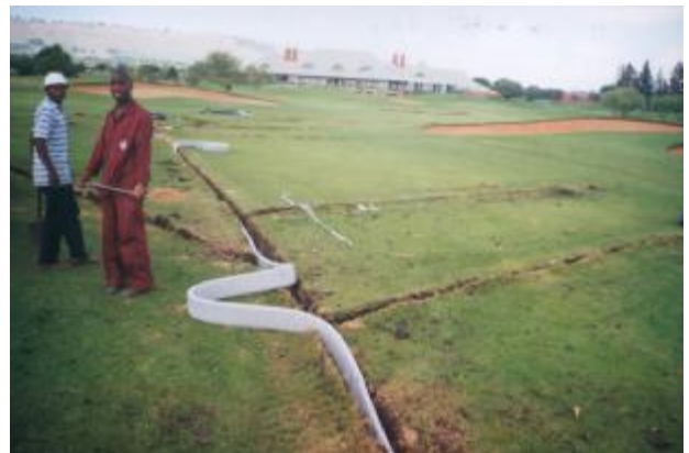
Placing MEGAFLO in herringbone trenches
