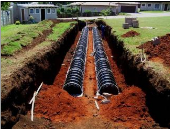
Infiltrator™ units placed in excavation
