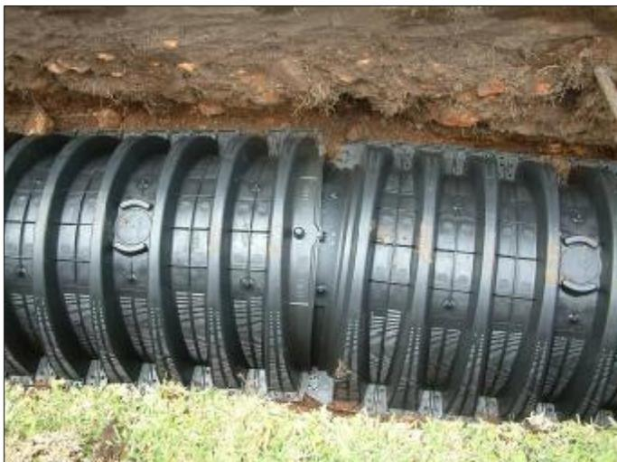
**Infiltrator™ Chambers** also permit the installation of inspection ports, in this case three, to monitor possible contamination of the system.
