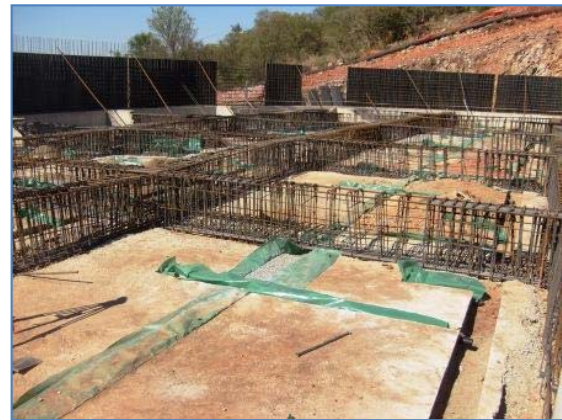
The grid system for leak detection
