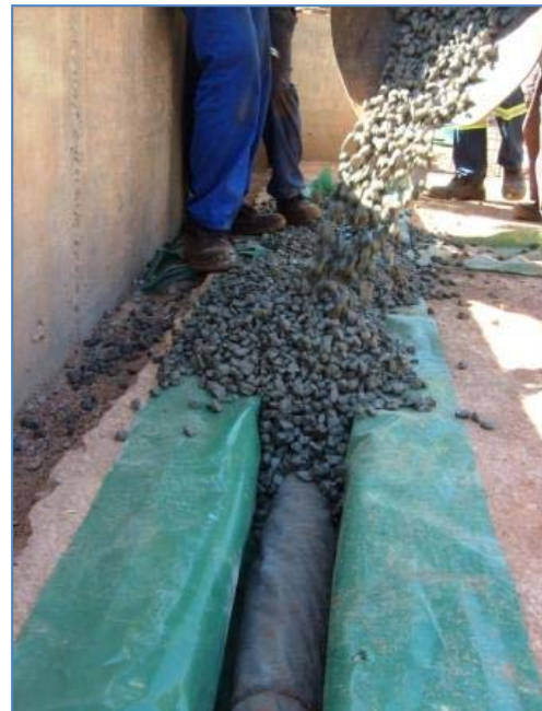
The bidim ® -wrapped Flo-Pipe ® is covered with no fines concrete
