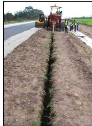
Digging the narrow trench
