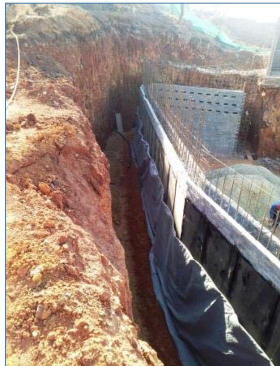
*The 3 m high retaining wall that required a drainage system*
