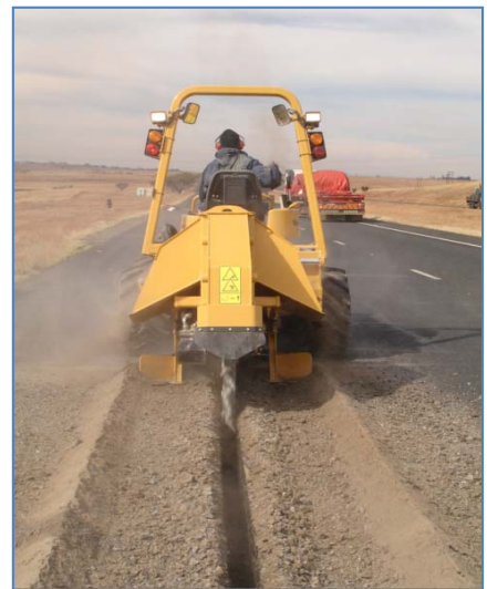
Rock saw digging the trench
