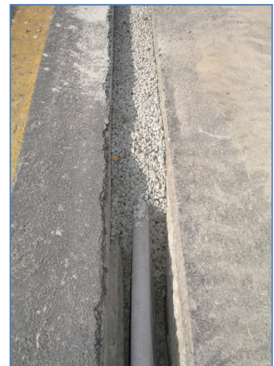
Megaflo™ installed with backfill
