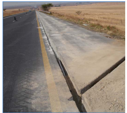
Section of N3 with before final asphalt layer applied
