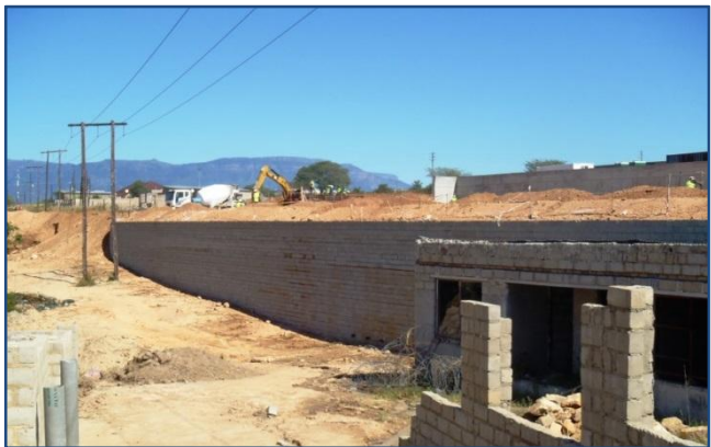
Part of the reinforced retaining wall at the Acornhoek Mall.
