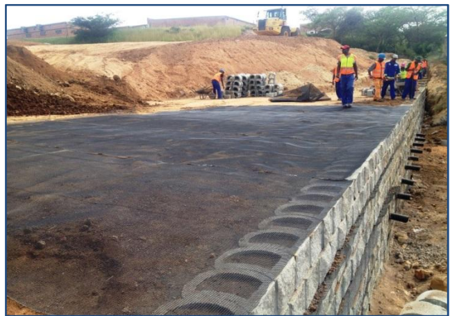
Miragrid GX 75/75 grid used to reinforce the retaining wall.
